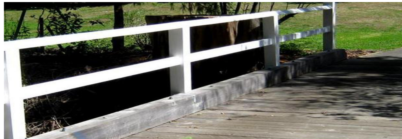
Figure 20– Bridge boards should be closely spaced - top rail should be angle cut.
