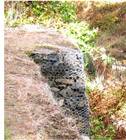
Figures 33, 34, 35 and 36 L-R: Creek walls: Dry stone and rubble creek walls are significant and contributory heritage features in themselves and are an integral part of Walhalla's heritage landscape. These should be conserved. Gabions and treated pine treatments are not.
