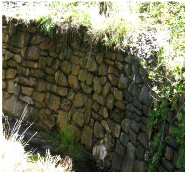
Figures 33, 34, 35 and 36 L-R: Creek walls: Dry stone and rubble creek walls are significant and contributory heritage features in themselves and are an integral part of Walhalla's heritage landscape. These should be conserved. Gabions and treated pine treatments are not.
