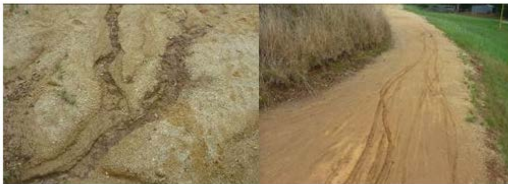
Figure 16: Water and run off damage to track
