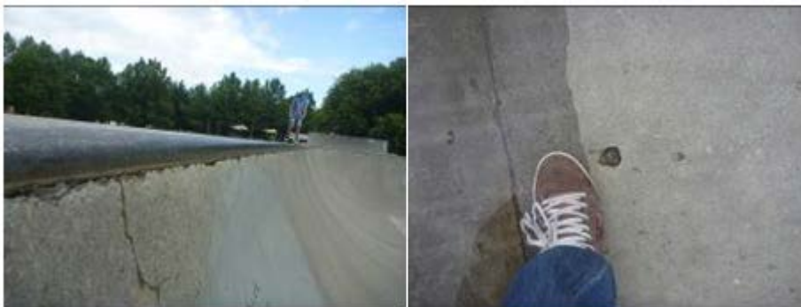
Figure 18: Views of some cracking and anti-graffiti paint and pock marks on the park
