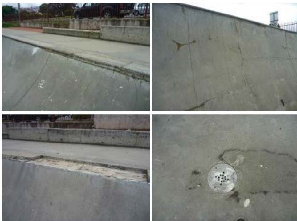
Figure 29: Views of the damaged/removed coping and existing drainage grate.
