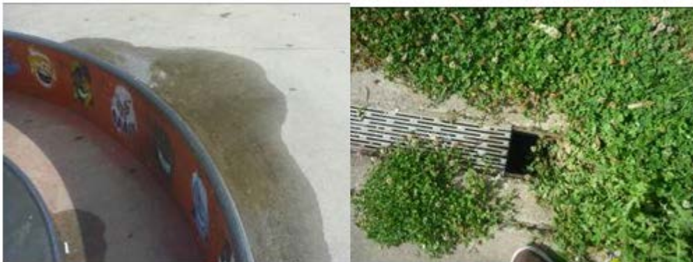
Figure 14: Images showing water ponding and damaged drain
