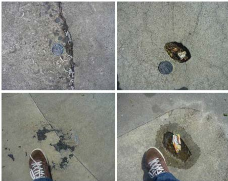
Figure 11: Views of various holes, spalling, burned plastic damage and cracks
