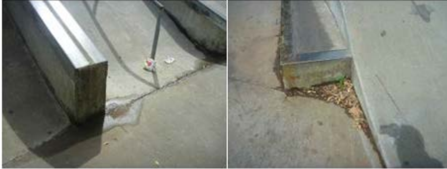
Figure 20: Views of water pooling and build-up of leaf litter
