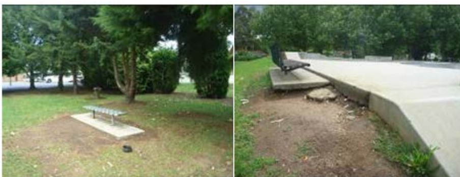
Figure 19: Views existing seating and wear around bases
