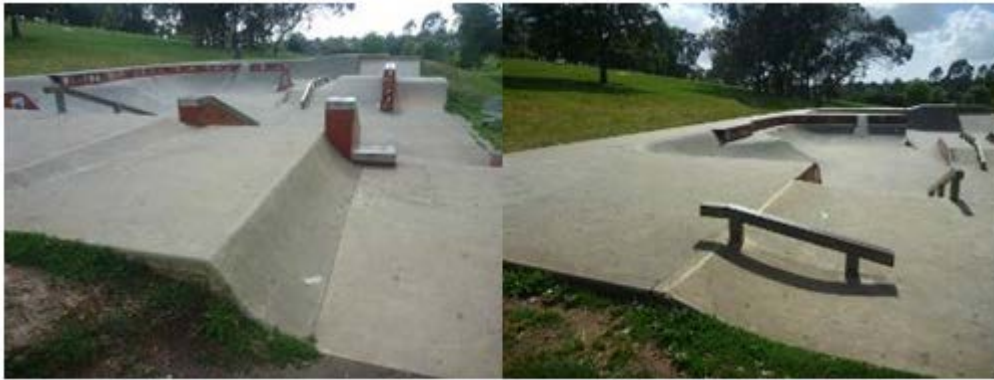
Figure 12: Steep transition between landings and low short rail
