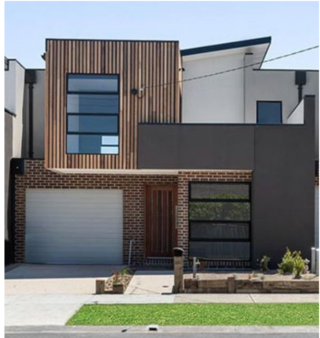
Example of a typical contemporary townhouse where the garage design does not visually dominate the dwelling facade.
