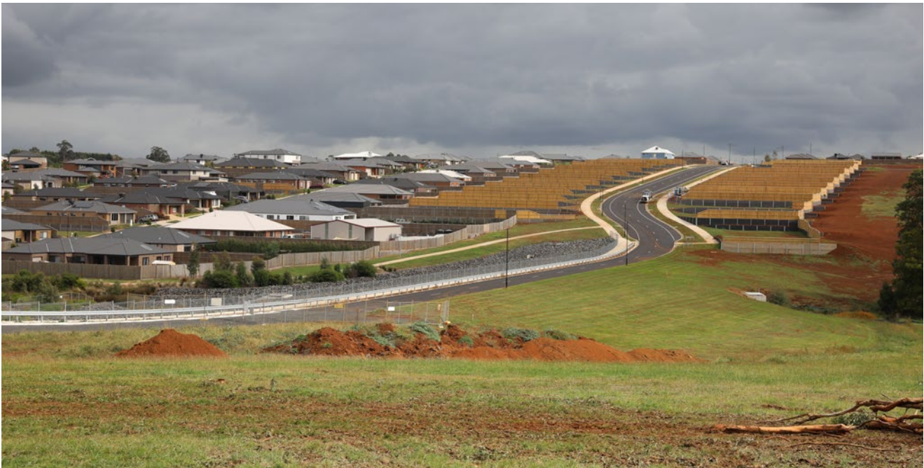
New residential housing being delivered in Warragul.
