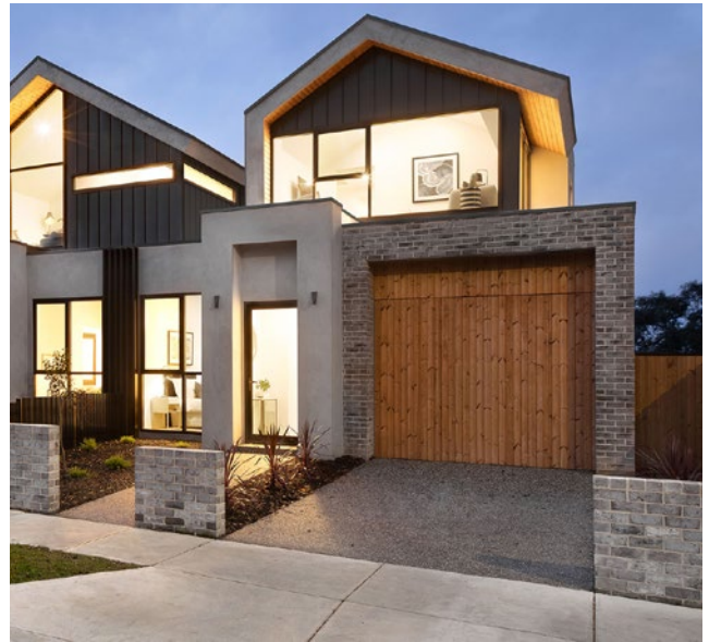
Example of a contemporary townhouse with a well articulated front entrance.
