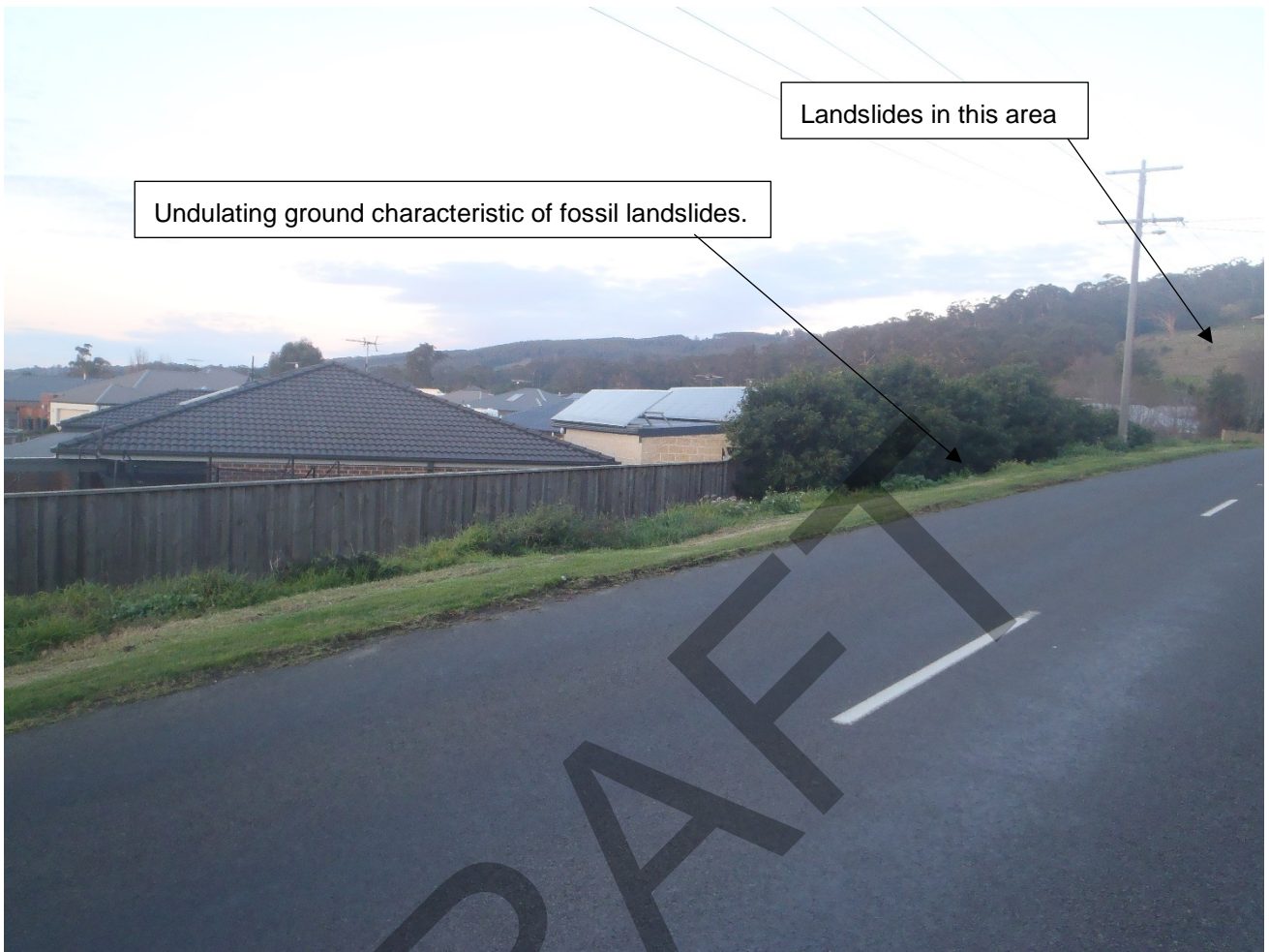
Figure 13: Residential development near foot of landslides at Trafalgar, Thorpdale-Trafalgar Road.
