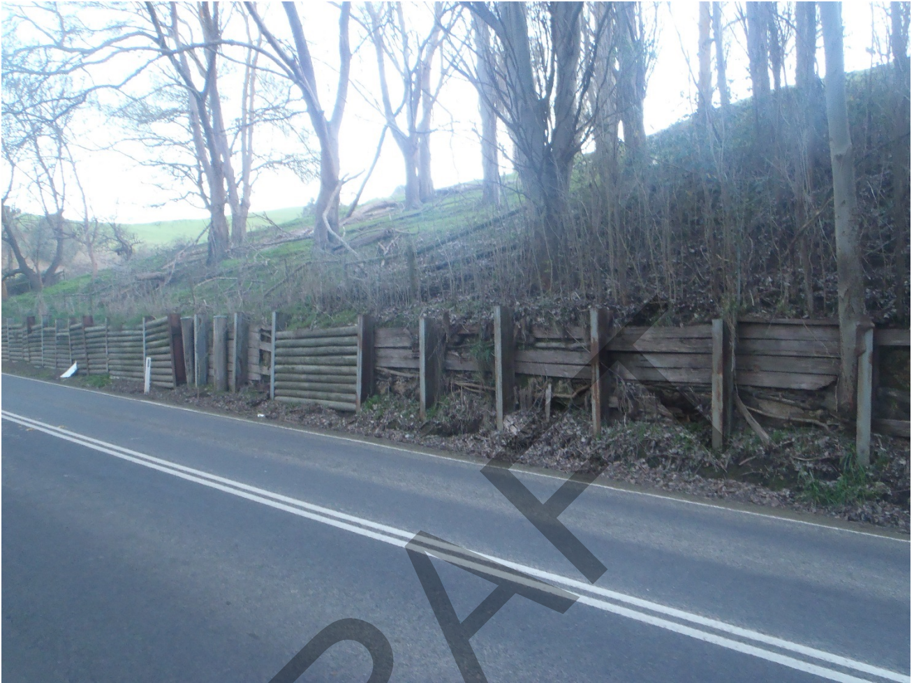
Figure 12: Examples of retaining walls supporting earthflows on the Thorpdale-Trafalgar Road.
