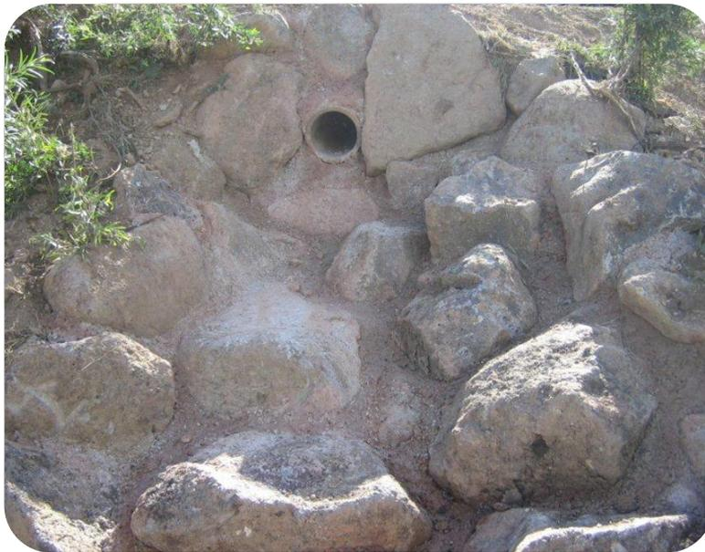
**Figure 19. Rocking of culvert outlet absorbs the energy of run-off and traps sediment. Photo courtesy of Nillumbik Shire Council.**
