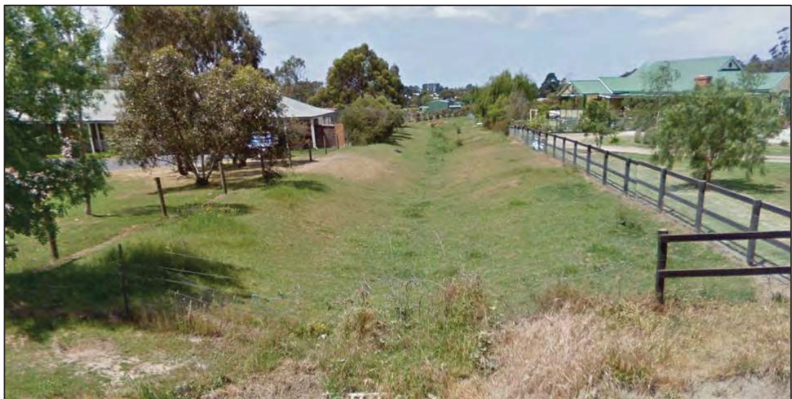
Figure 5.1 Example of open drain / floodway
