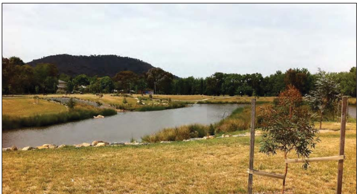
Figure 5.2 Example of retarding basin (including optional permanent pond / wetland)
