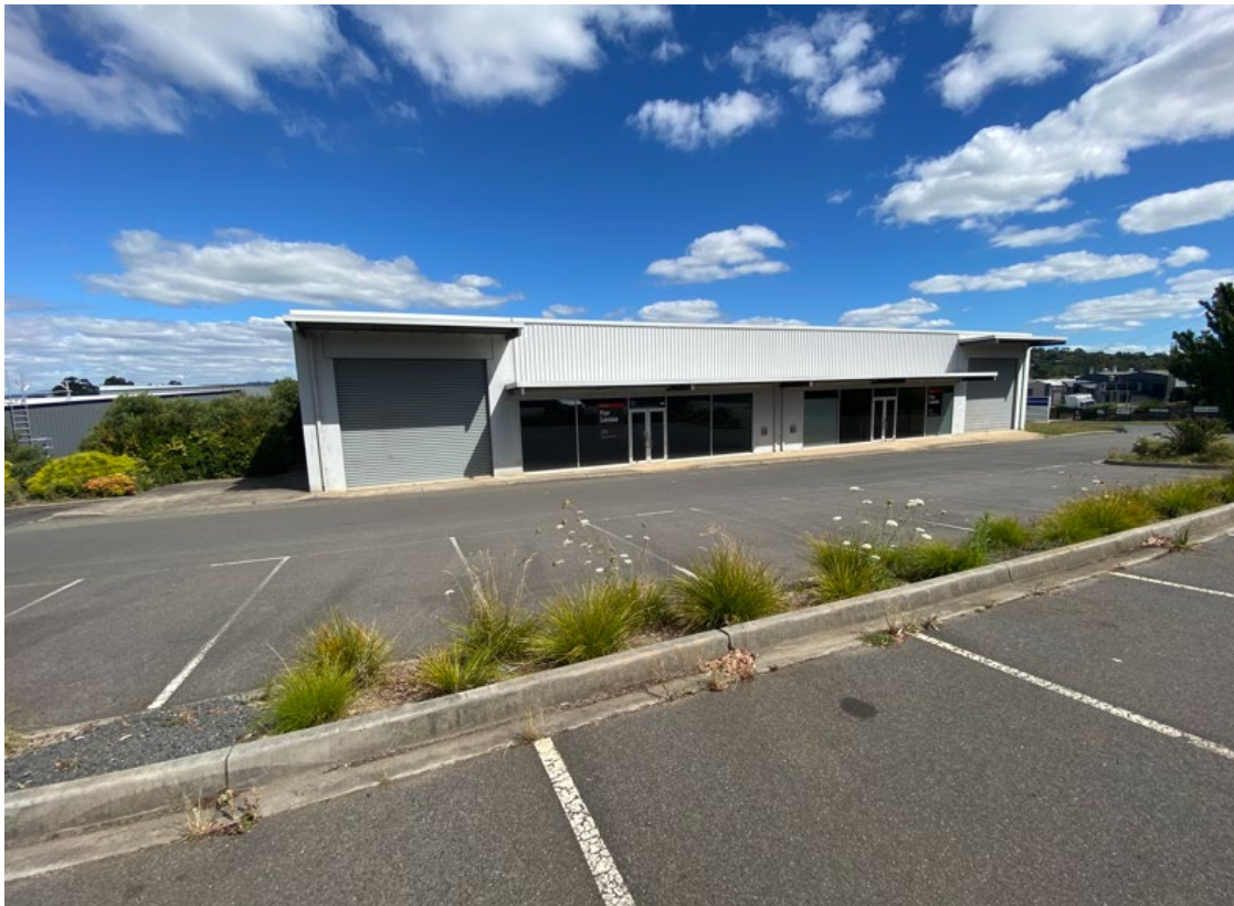
Figure 4: View of the subject site frontage Unit 1 and adjoining property Unit 2
