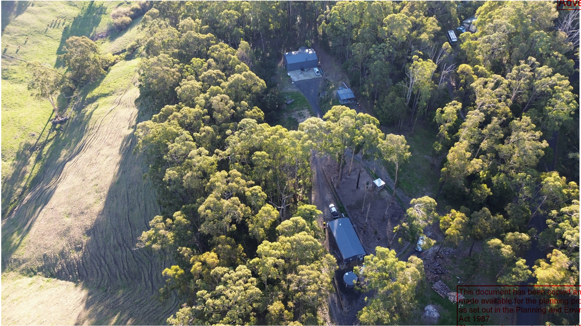
Photo 5 – Aerial photo of the slope of adjacent property
