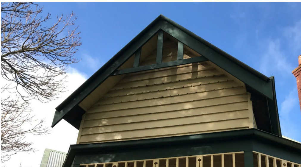
Figure 13 Detail of original gable ends and bargeboards. Note notched weatherboards in gable ends. Source: Plan Heritage, 2020
