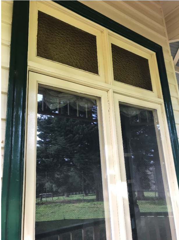
Figure 14 Original window in north west projecting gable - note coloured textured glass remaining in upper panes. Source: Plan Heritage, 2020
