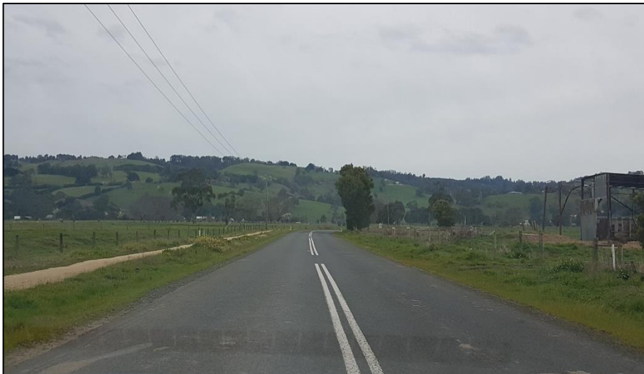
FIGURE 5: YARRAGON-LEONGATHA ROAD FACING SOUTH
