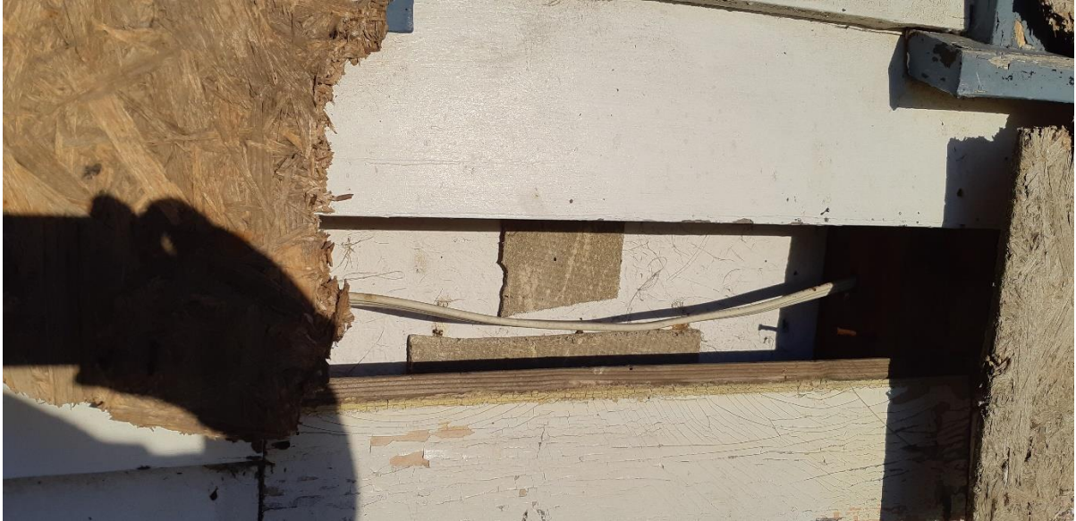
Plate 3: 63 Yarragon-Leongatha Rd, Yarragon (Asbestos Containing Material (ACM) located within the walls of the dwelling)
