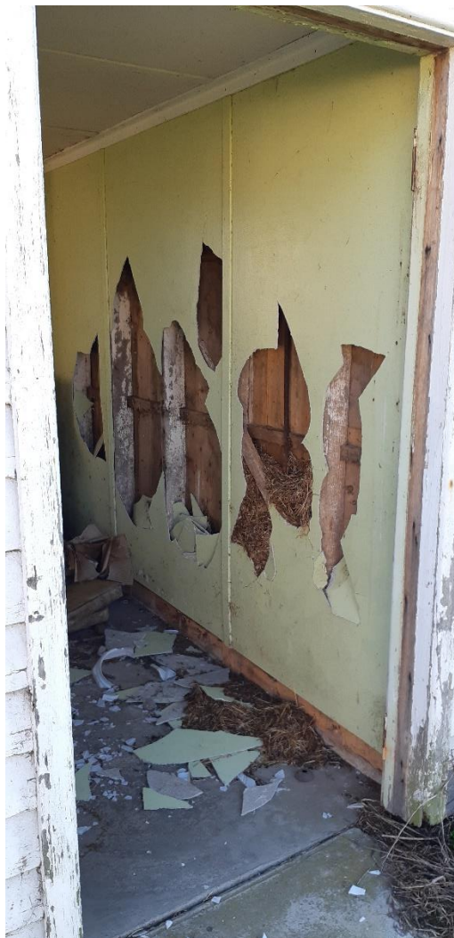
Plate 4: 63 Yarragon-Leongatha Rd, Yarragon (structure to the rear of abandoned house- walls and general condition of the building was poor). ACM within wall linings and on floor.
