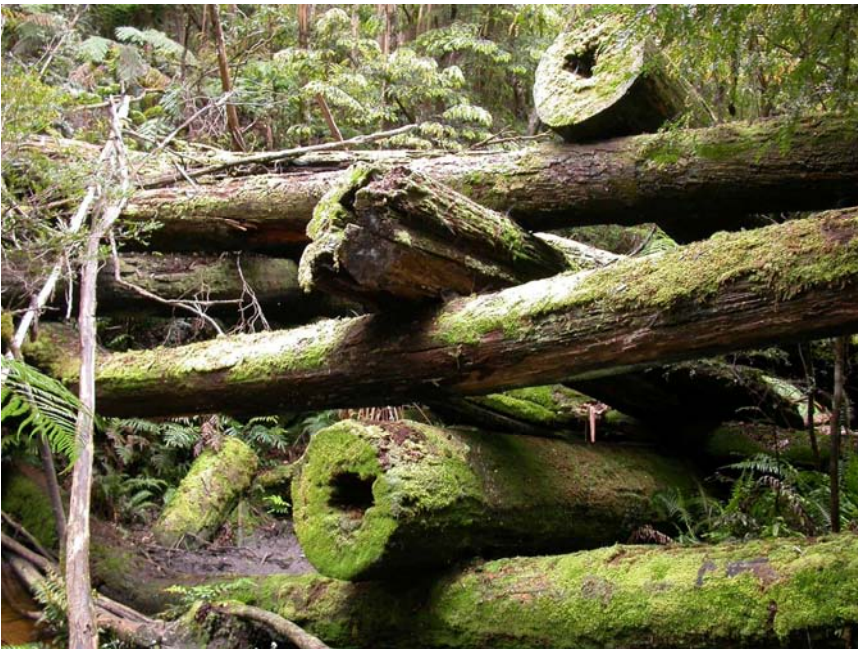
New Federal Mill bridge remnants 2005
