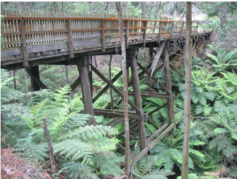
Old timber road-over-rail bridge at Bloomfield Road, Crossover
