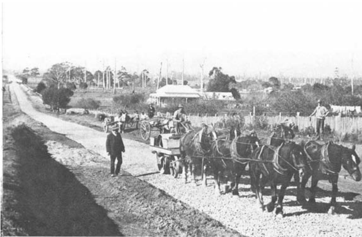
Construction of the main Gippsland Road [Princes Highway]
