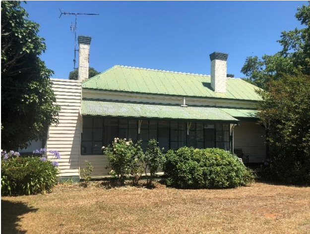
Plate 3: North elevation of 14 Tarago Court, Warragul showing sleepout built into veranda (Source: Ecology and Heritage Partners Pty Ltd January 2019)
