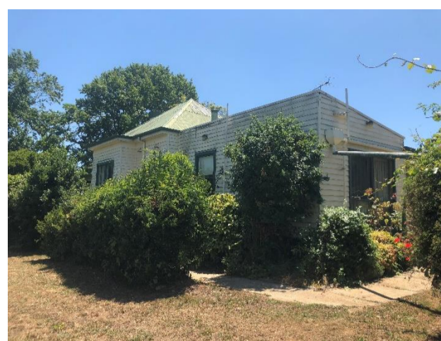
Plate 2: South east elevation of 14 Tarago Court, Warragul (Source: Ecology and Heritage Partners Pty Ltd January 2019)
