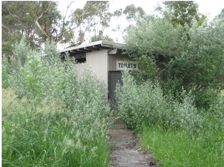
Existing disused former pony club's toilets and sheds to be removed
