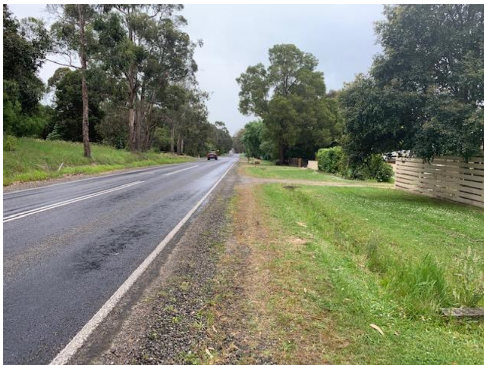
Photo 1 Subject land - existing access
