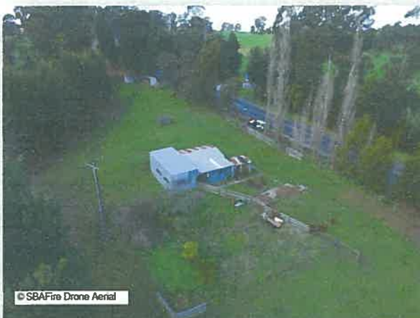
3 View southeast above dwelling site to sheds and entry gate
