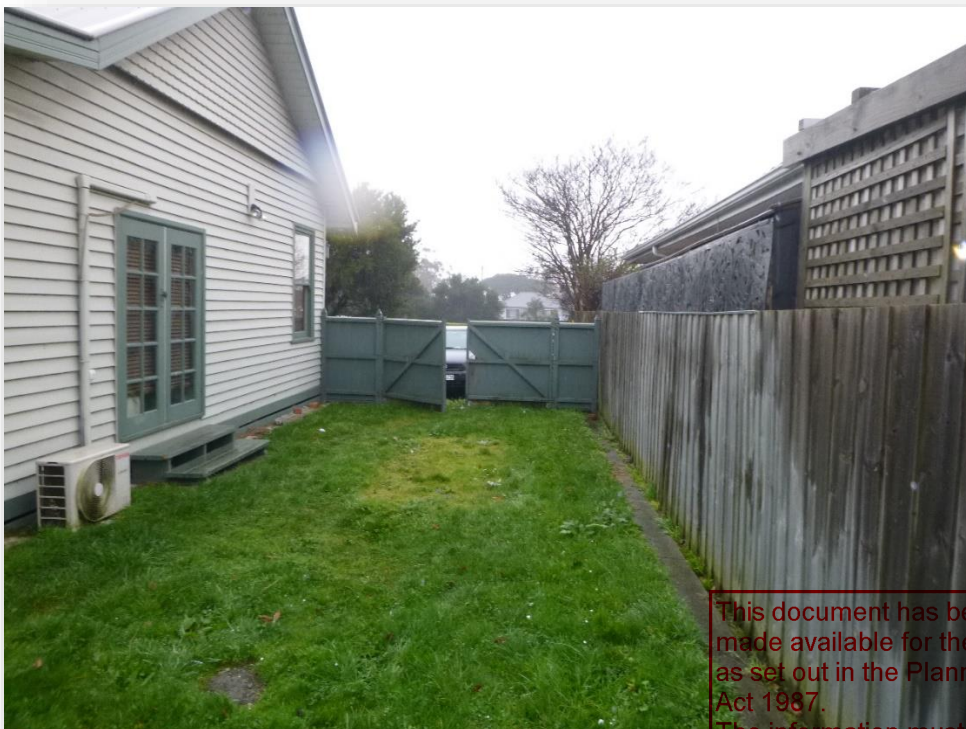
Image 6: View of existing access way – to be concrete paved and new carport to be installed.
