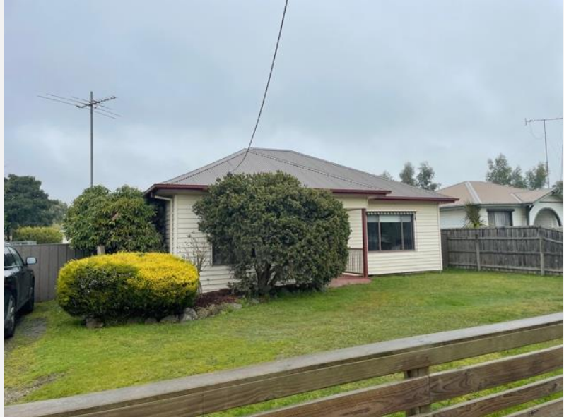
Typical residential development along Princes Highway.
