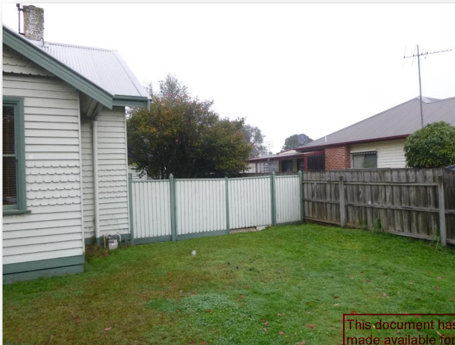
Image 8: View existing wing fence – to be removed and new access way to be installed for second dwelling.
