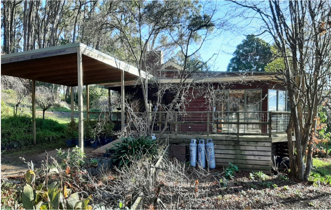
IMAGE 11 – Eastern view of the existing dwelling.
