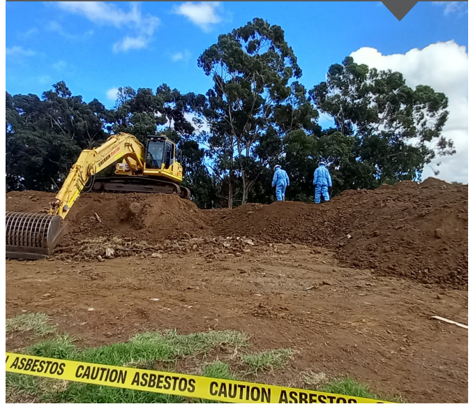
Critical asbestos abatement works underway under close supervision by hygienist professionals.
