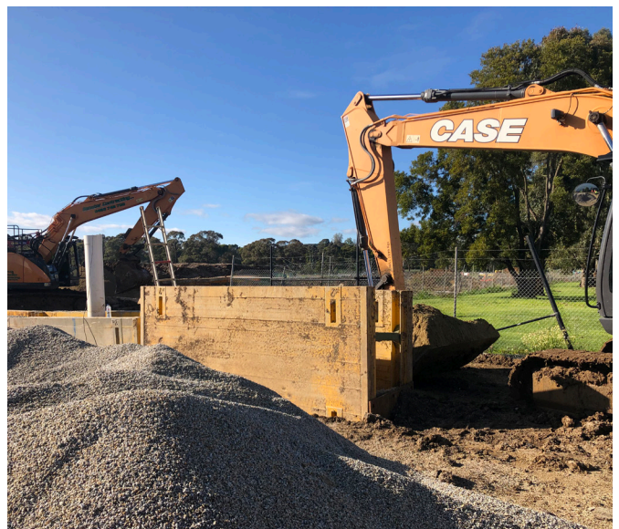
Sewer realignment works being undertaken by O'Brian Plumbing on behalf of Kubale Construction.
