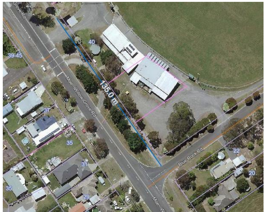
Figure 6 Footpath in front of the Recreation Reserve
