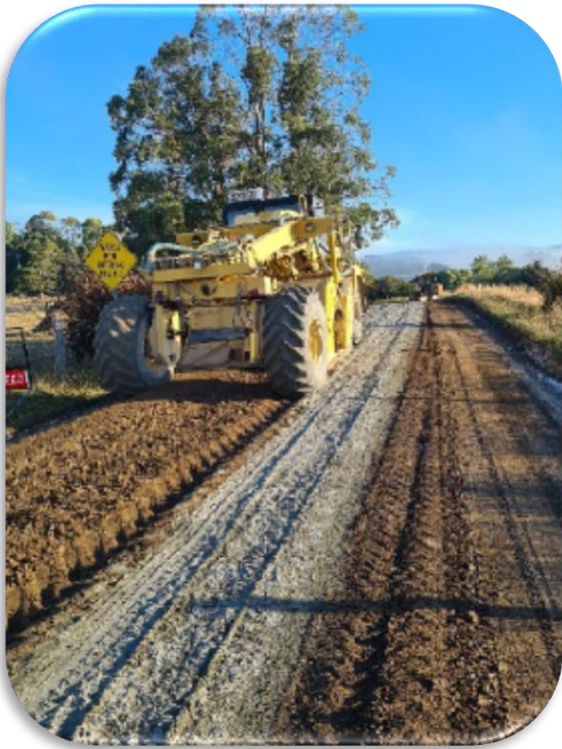
Neerim East Road – Mixing Work
