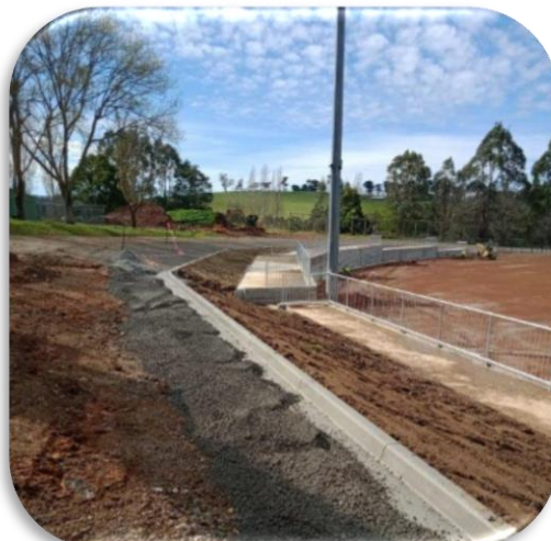
Retaining wall at Neerim South Oval
