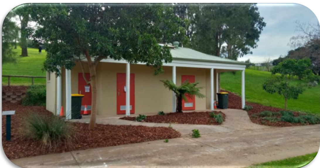
Drouin Civic Park Toilets
