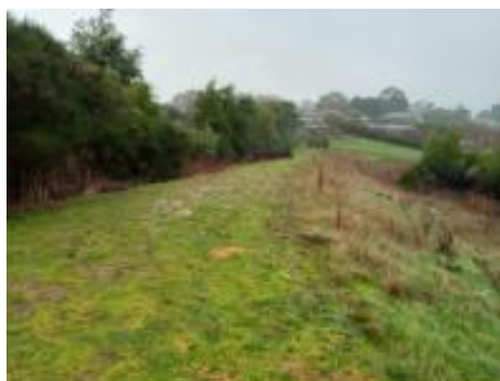
Bull Swamp Creek Dam Wall
