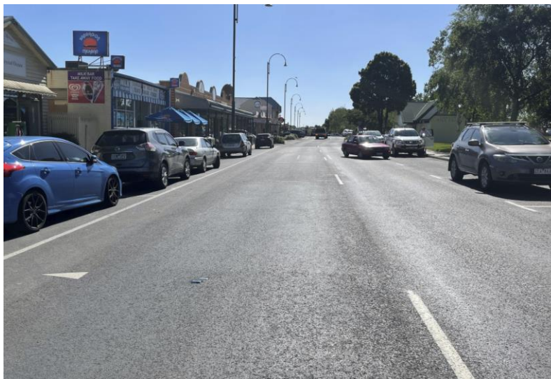
Figure 2.4: Princes Highway service road looking west
