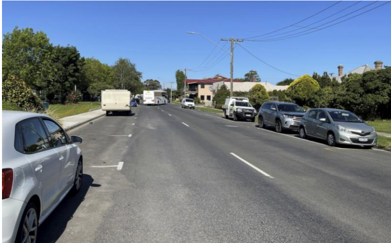
Figure 2.3: Princes Highway service road looking east
