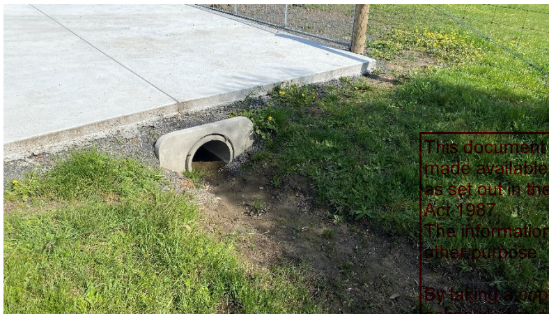
PHOTO 11 – EXISTING CULVERT UNDERNEATH CROSSOVER PROVIDING ACCESS TO SITE
