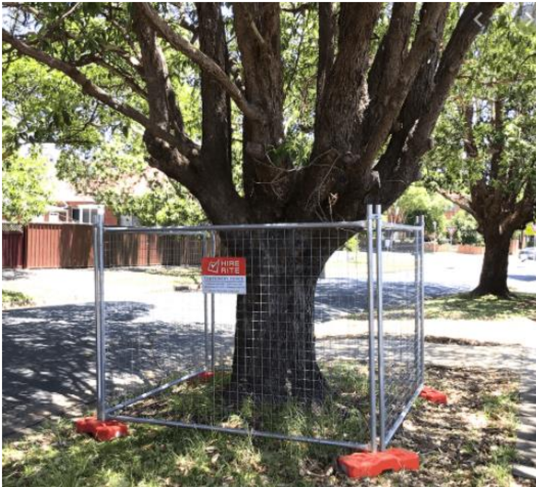
Figure 3: Example of public tree protection zone fencing
