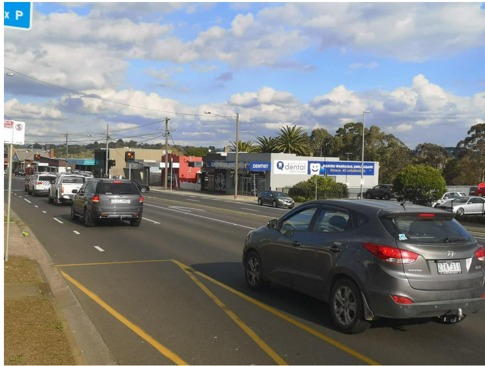
EXISTING PERSPECTIVE VIEW #01 - EASTBOUND TRAFFIC
