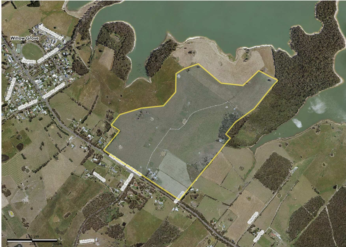
Figure 1: Aerial image showing the site.
