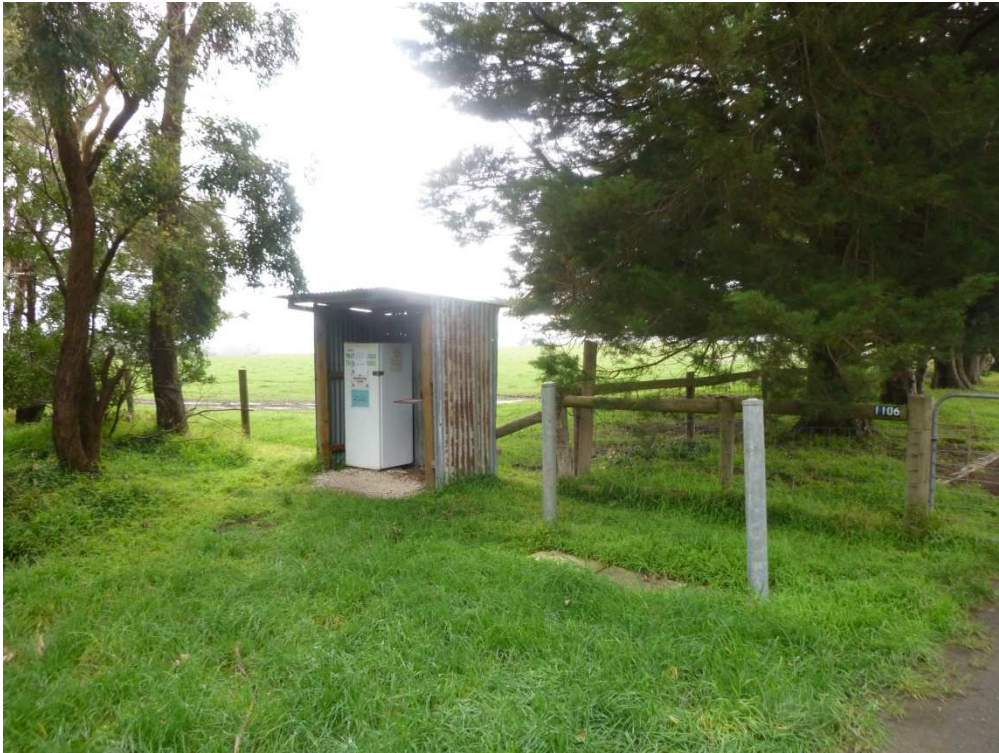
Facing north – Existing road-side trading shelter- this will be demolished and re-located within the property boundaries (refer to attached architectural plans for proposed location).
