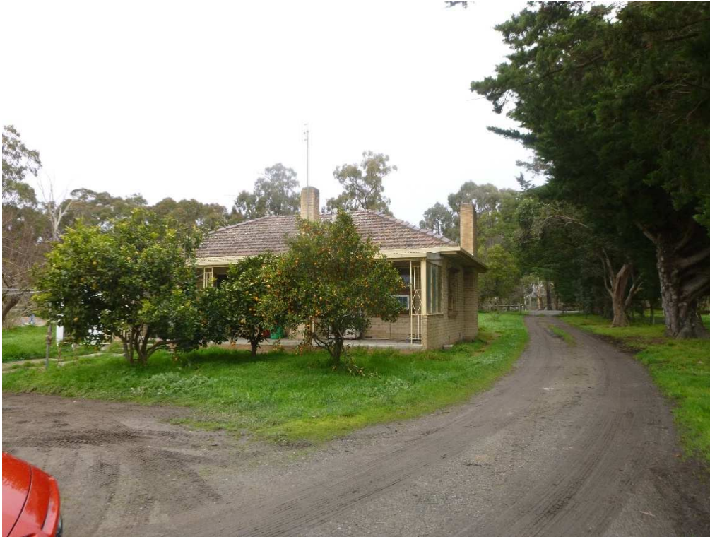
Facing south-west – looking towards Moe-Willow Grove Road.
