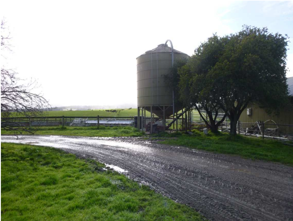
Facing north-east – existing silo being used for the storage of feed for the poultry before being distributed to the hens on-site.
