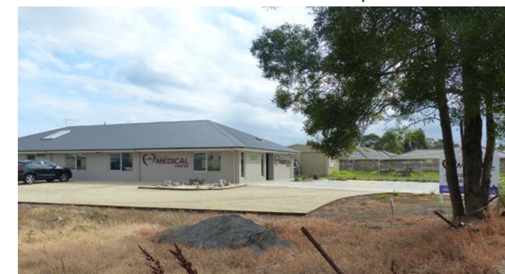
Contemporary medical centre with associated car park
