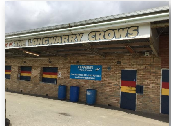
The existing AFL/Cricket player change rooms and supporting amenities are aged and do not meet peak sporting body preferred facility standards for a 'Local' level facility.
