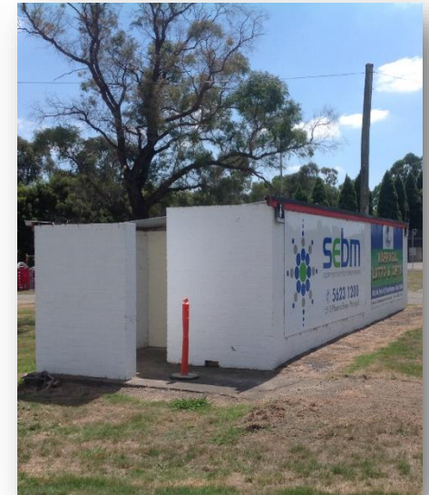
The above public toilet facility receives high levels of use but is aged, inadequate and requires replacement.
