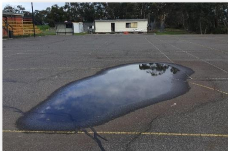
Netball Court number one's uneven surface presents a risk management and safety concern for users and is often subject to pooling of water in 'sunken areas'.
