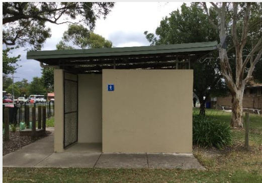
The frequently used public toilet facility at the Reserve's entrance is aged, inadequate and requires replacement.
