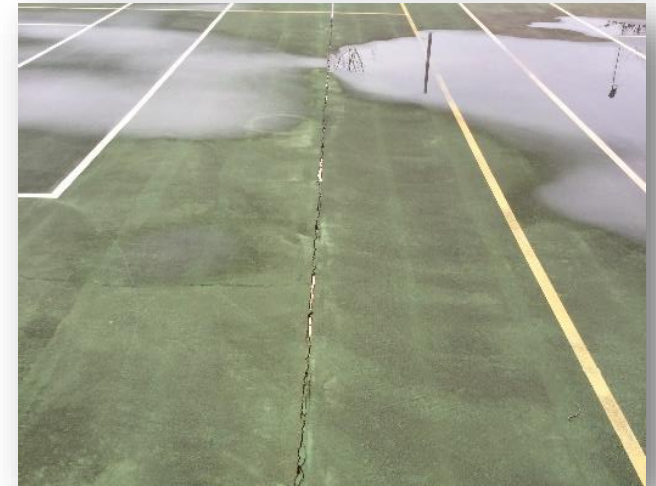
The aged multi-purpose netball/tennis court surfaces are cracking, uneven and subject to water pooling.
