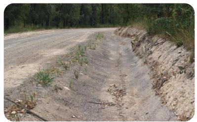
Figure 14. Cement-treated table drain on Rankines Road, Strathewen.
