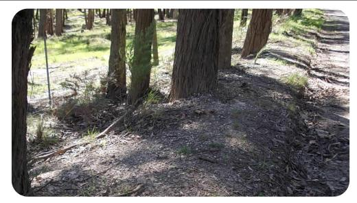
Figure 9. Excess materials should not be stockpiled against the base of a tree.
