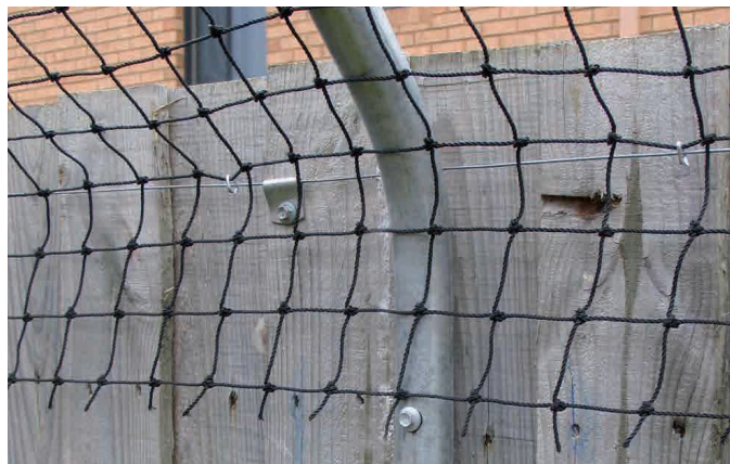
Figure 6: Netting fixed to fencing with wire
