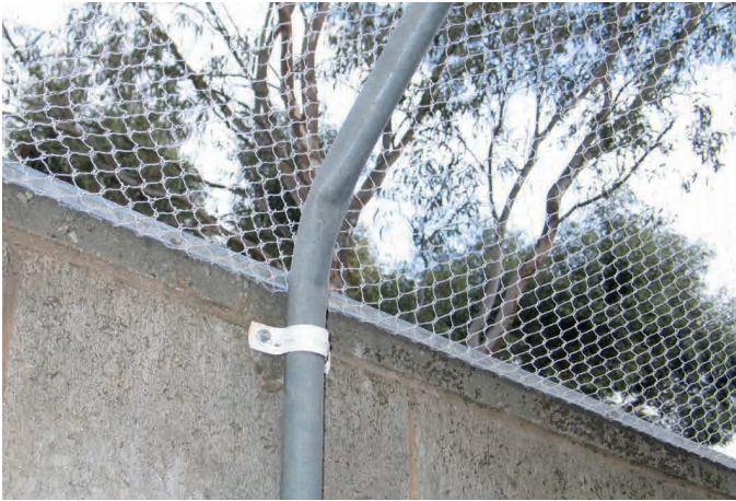
Figure 7: Netting fixed to fencing with brace
