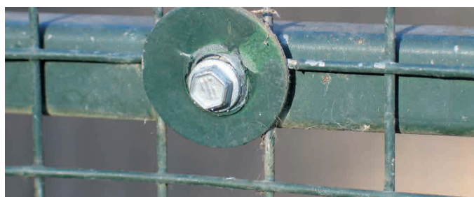
Figure 5: Fixing light mesh
