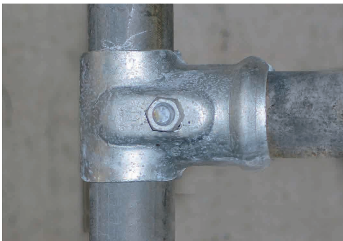
Figure 8: Prefab pipe fitting
