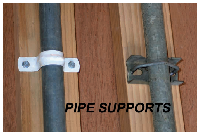
Figure 4: Fixing support pipes
