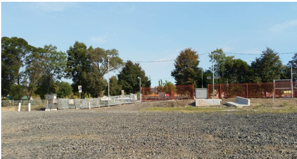
Figure 18 Existing pedestrian access from the north to the railway station
