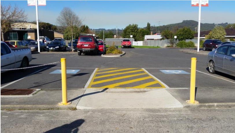
LOCATION 2 MCCROREY EAST CAR PARK NO. SPACES: 2 OFF STREET ISSUE: NO BOLLARD
